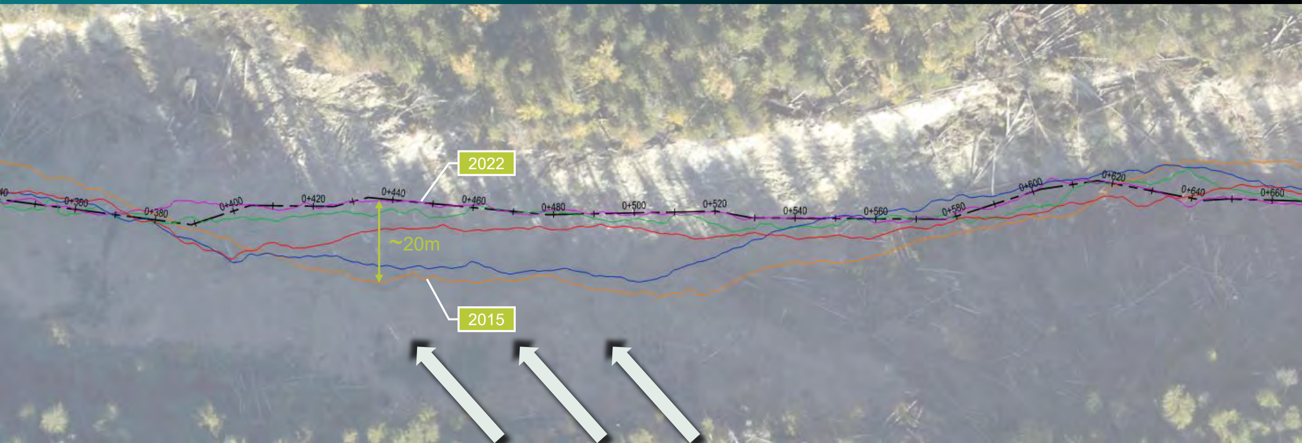
Football Field Landslide (FFL)
